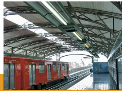
Subway station with daylight and additional artificial lighting
