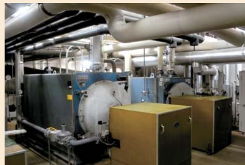
The school heating system, outdated and in need of renewal. As it was operated by the local energy utility, the system could not be upgraded in the ECO-Watt project.
