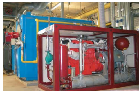
New boiler and CHP plant in the solar energy and economy project, Europa school, Cologne
