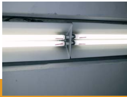
Inefficient T12-tubes with magnetic ballast
